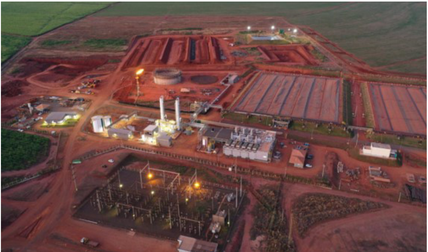
Aerial photo of the biogas plant at the Bonfim plant.
