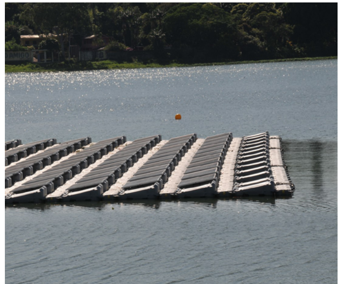
Floating solar power plant near Billings reservoir banks.
