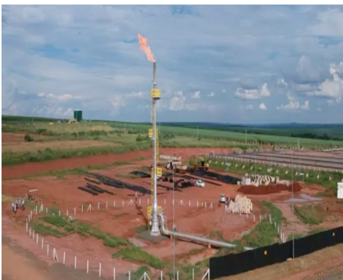
Flaring System at Bonfim Biogas Plant.
