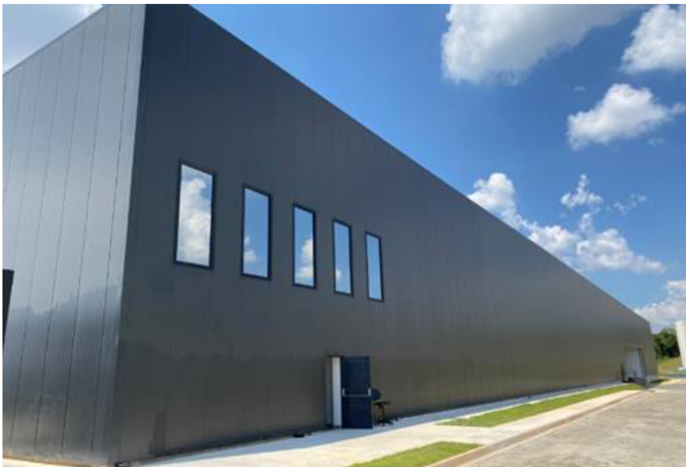
Parafix's Industrial Warehouse in Vinedo/SP with Steligence solution application.
