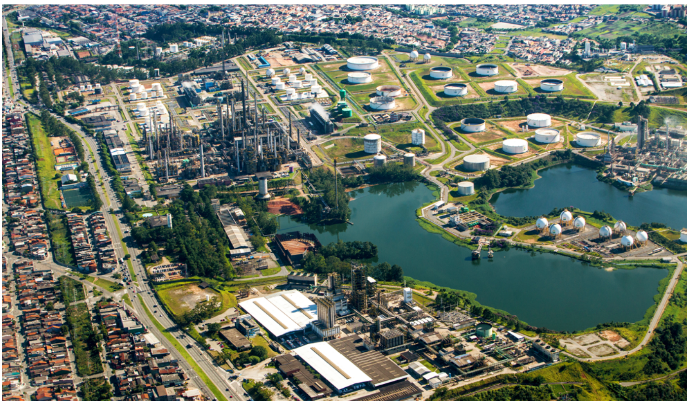
ABC Petrochemical Complex (Q3 and PE7 units).
