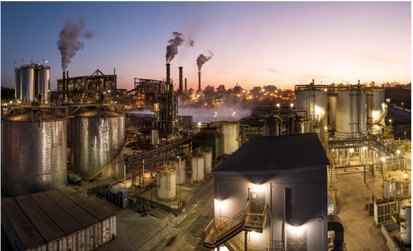
Aerial photo of the 2G ethanol plant installed at the Costa Pinto unit.
