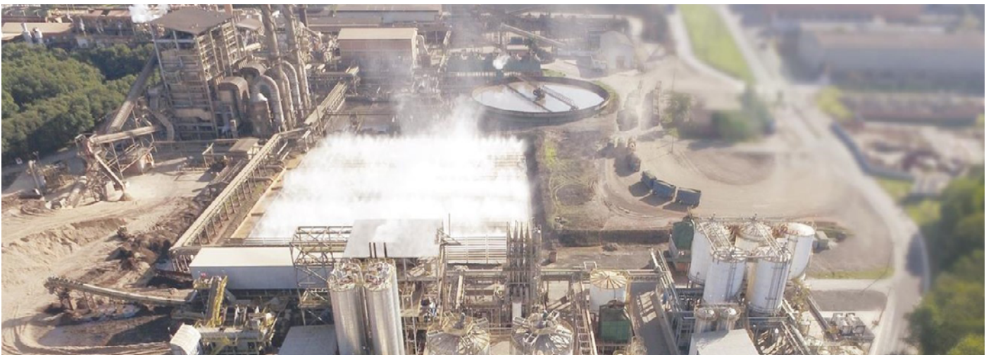
Aerial photo of the 2G ethanol plant installed at the Costa Pinto unit.
