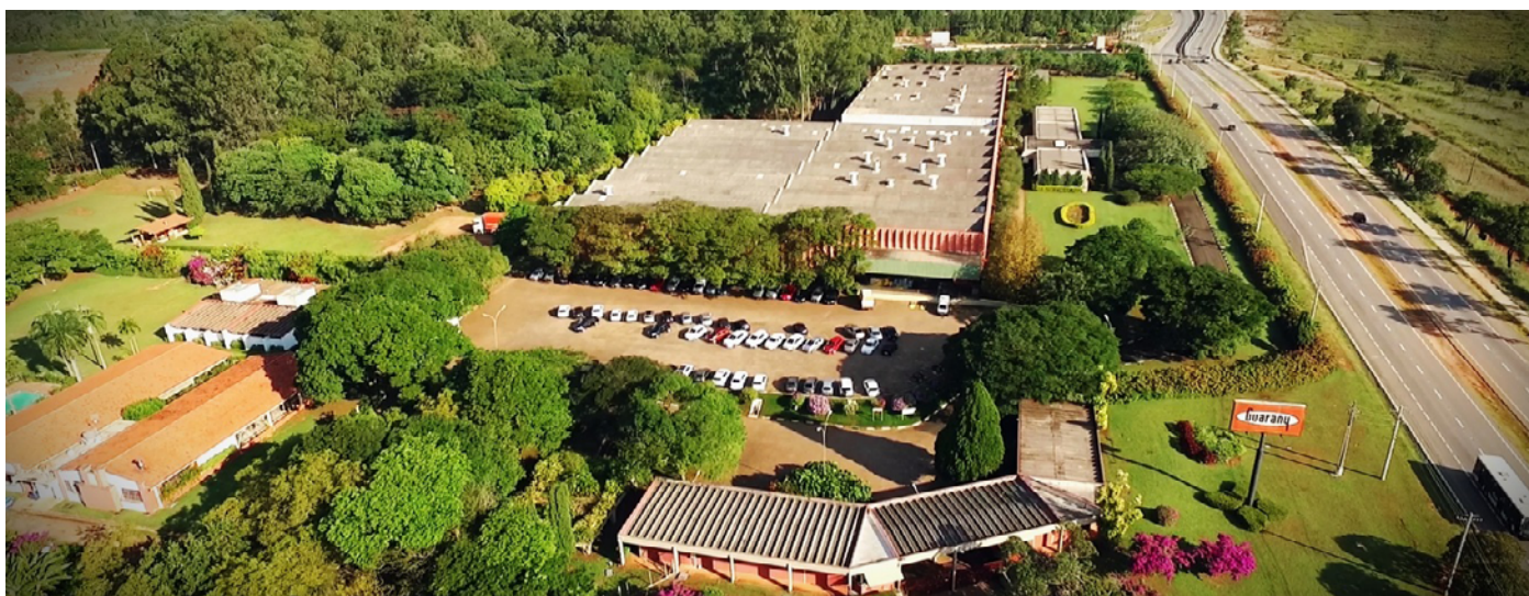
Guarany industrial facility in Itu.
