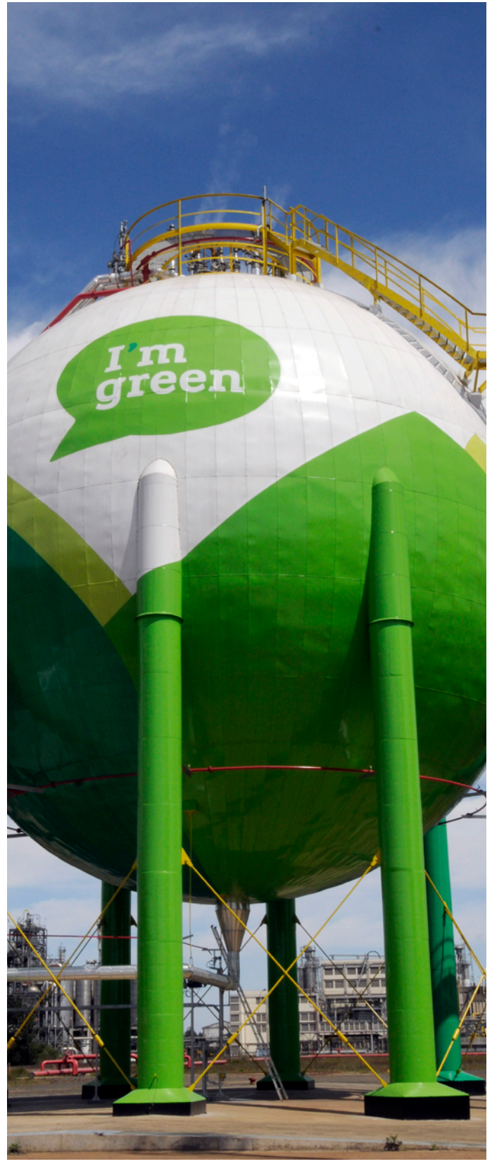
Green ethylene production at Triunfo, Rio Grande do Sul.
