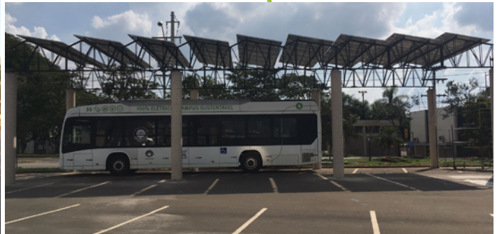
Completion of carport construction.
